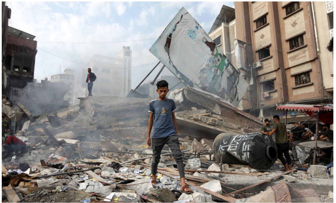
Palestinians inspecting damage to buildings and houses in Khan Younis following Israeli airstrikes, in the southern Gaza Strip on Oct. 10, 2023. | The New York Times
